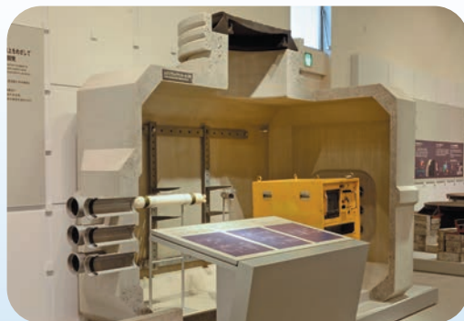
Manhole to pass through communications cable (model)
